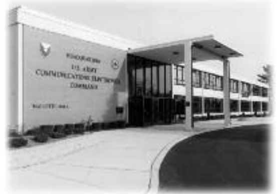
CECOM LCMC Headquarters - Building 1207. Renamed Mallette Hall in memory of LTG Alfred J. Mallette in 1996.
