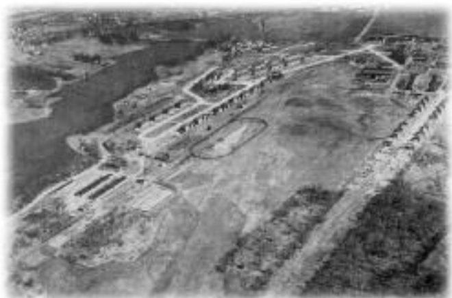
Fort Monmouth (January 1933). Construction underway on Field Grade and SNCO Quarters.
