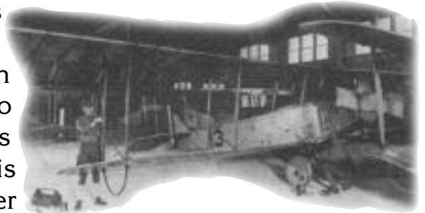
Camp Alfred Vail, NJ (Circa 1919). Radio Laboratory personnel installing radio equipment in Curtiss JN-4 (Jennys).
