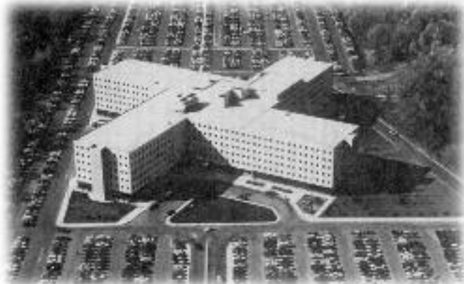
CECOM Office Building
